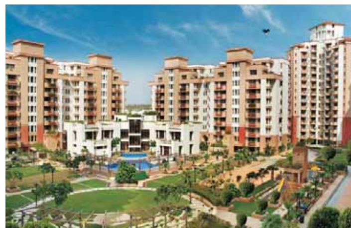
Vipul Gardens, Gurgaon
