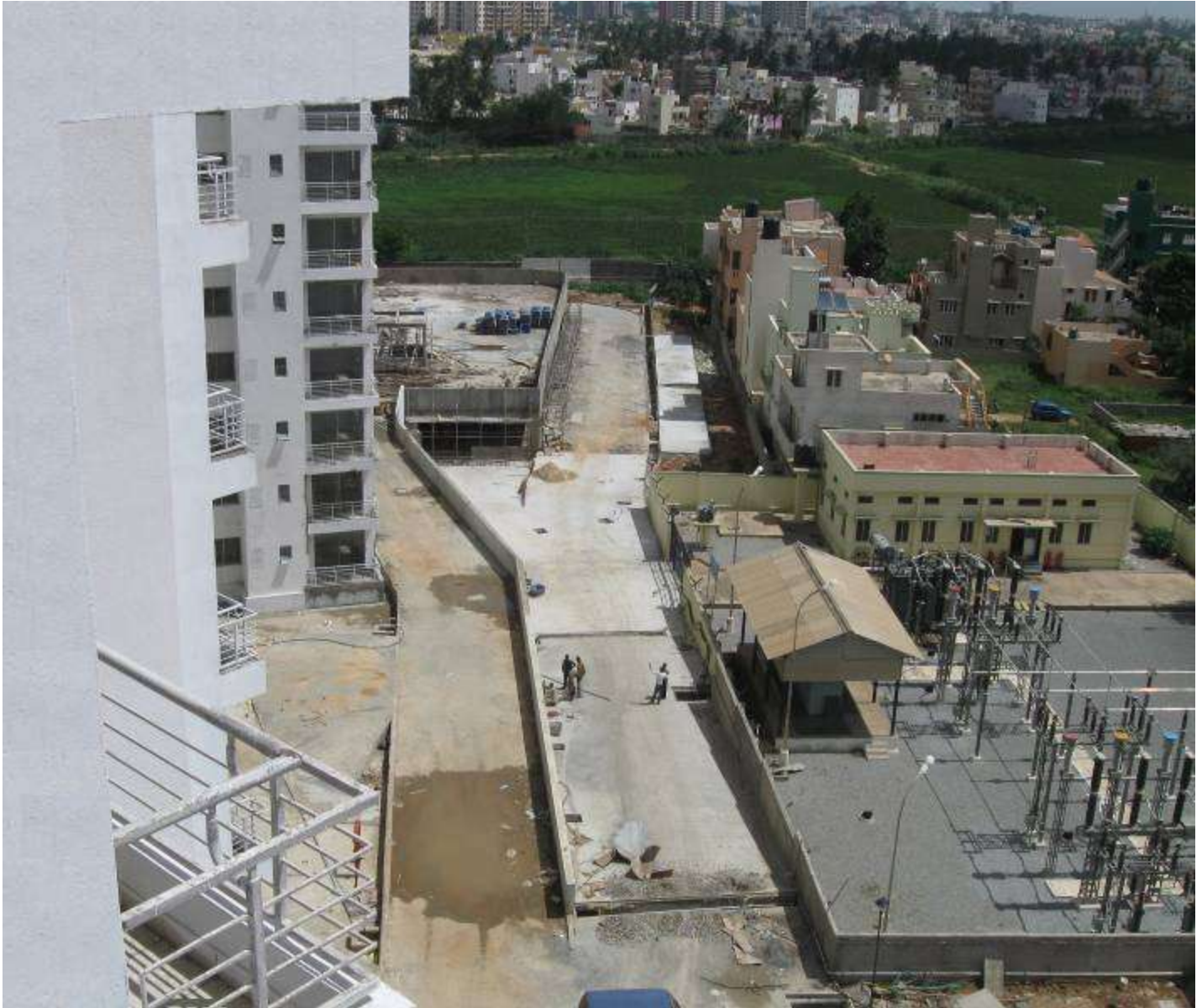
A view of the Rear Side of Phase 2 and the Sub Station
