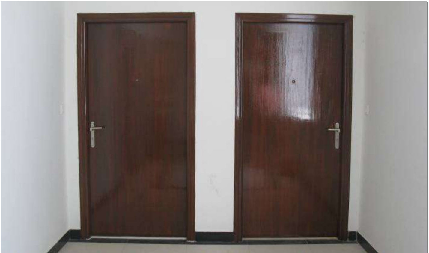
View of the Ready Units at B1 Block in Phase2
