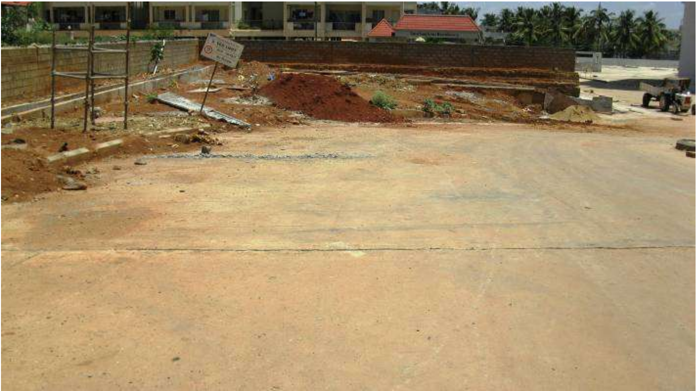
View depicting the Construction Progress of the Landscape at Entrance of Phase 2
