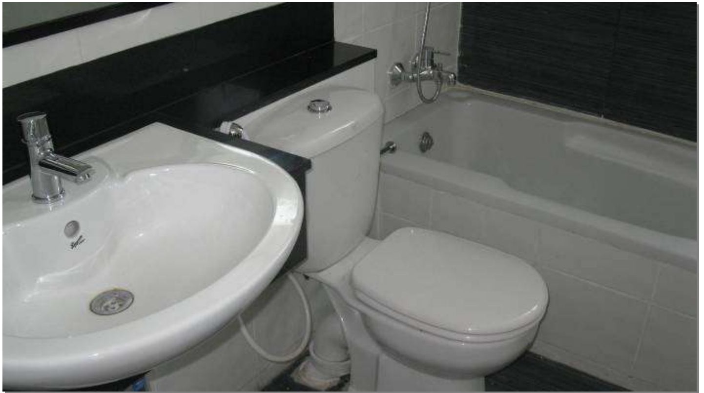
View of the Master Bathroom with all the fittings in a unit at Block B2
