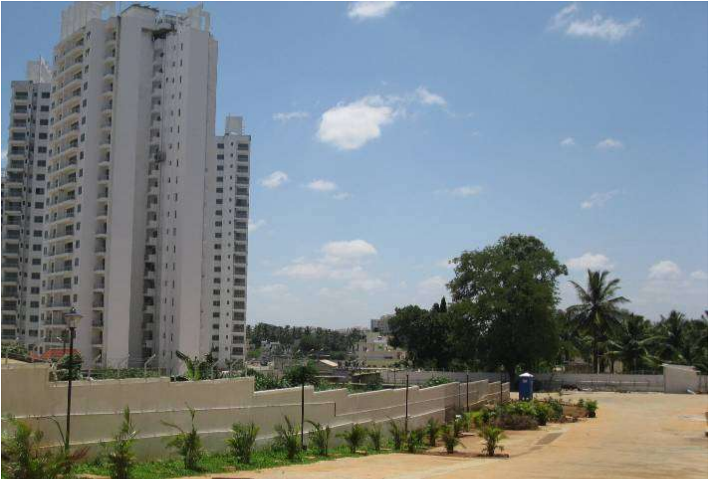
View of the road connecting to Phase2
