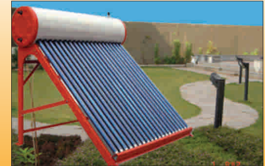
Solar water heating system.
