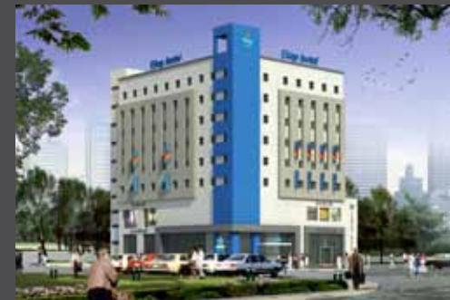
Accor Hotels Plot No-3, Sector Knowledge Park-III, Surajpur Kasna Main Road, Greater Noida City (Opening November 2011)
