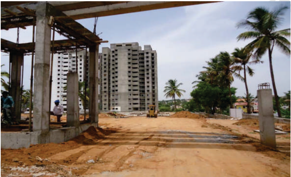
Road Formation Works
