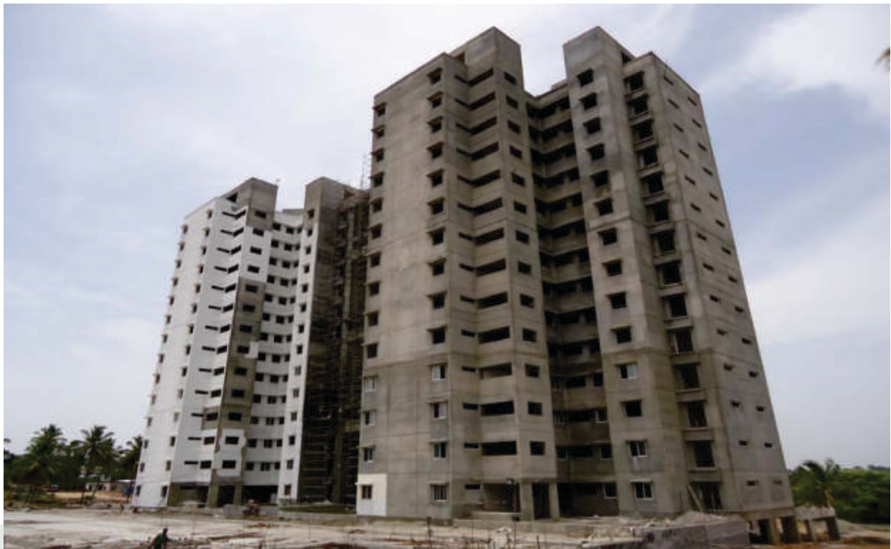
Both Tower C and D from North west Corner.
