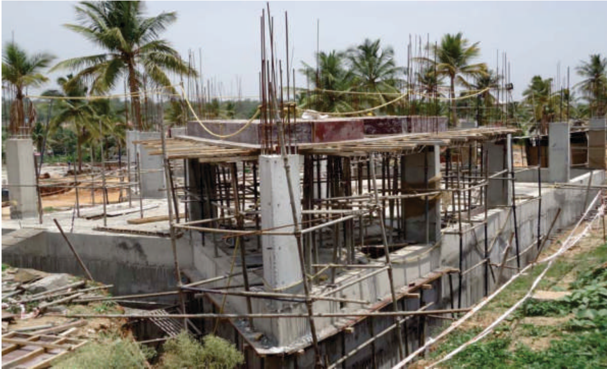
Club House First floor slab shuttering in progress
