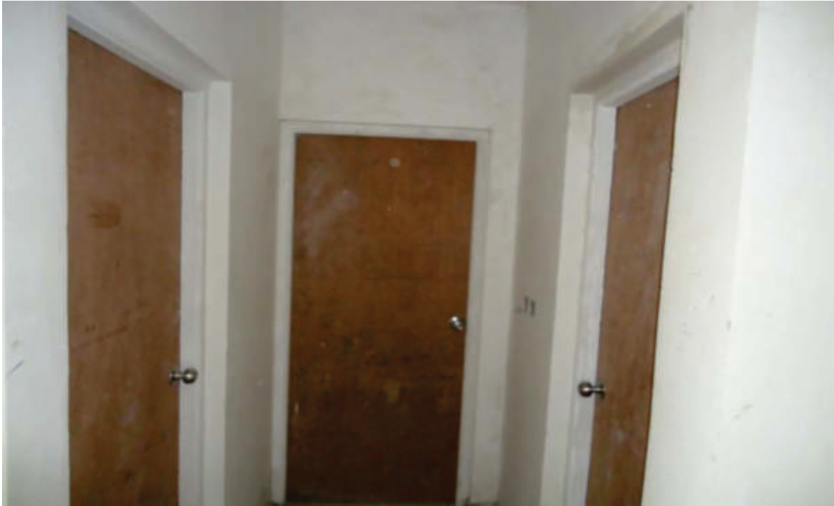
Fixing of Internal door shutters in progress.
