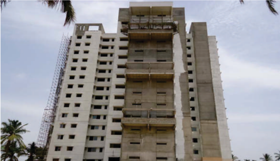
Tower C from East side.
