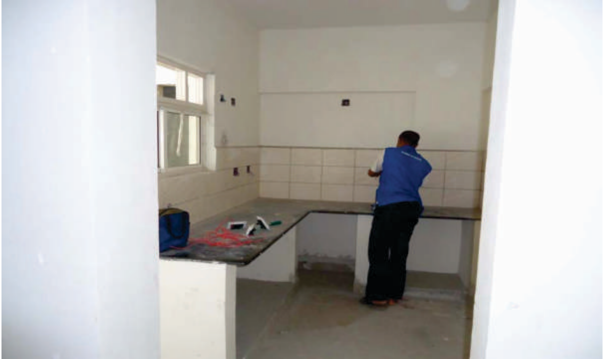
Internal wiring works are in progress
