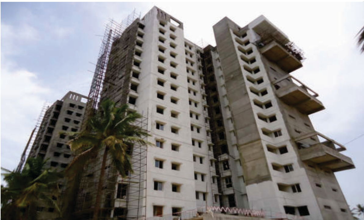
Tower C view from South East Corner.
