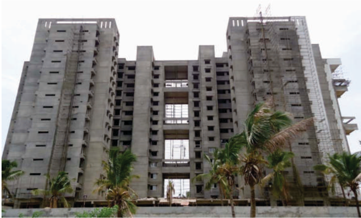
Both Tower C and D from South side.
