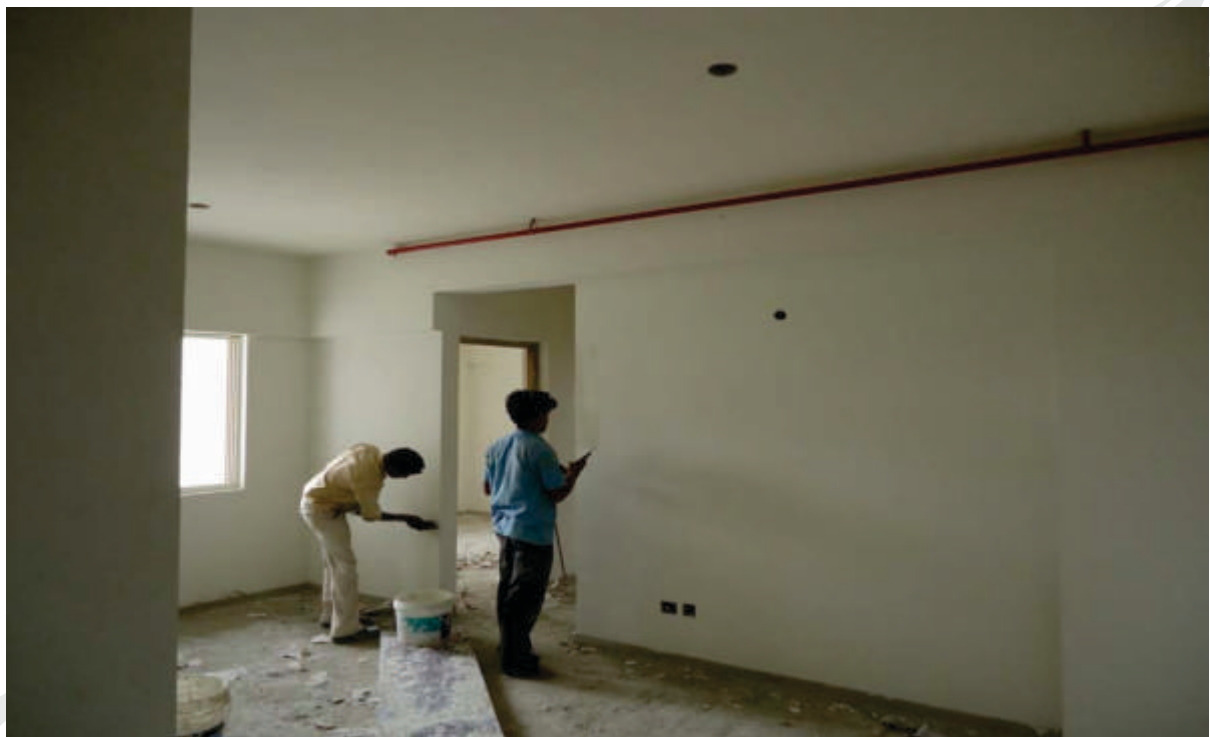
Internal Painting( Primary putty works are in Progress).
