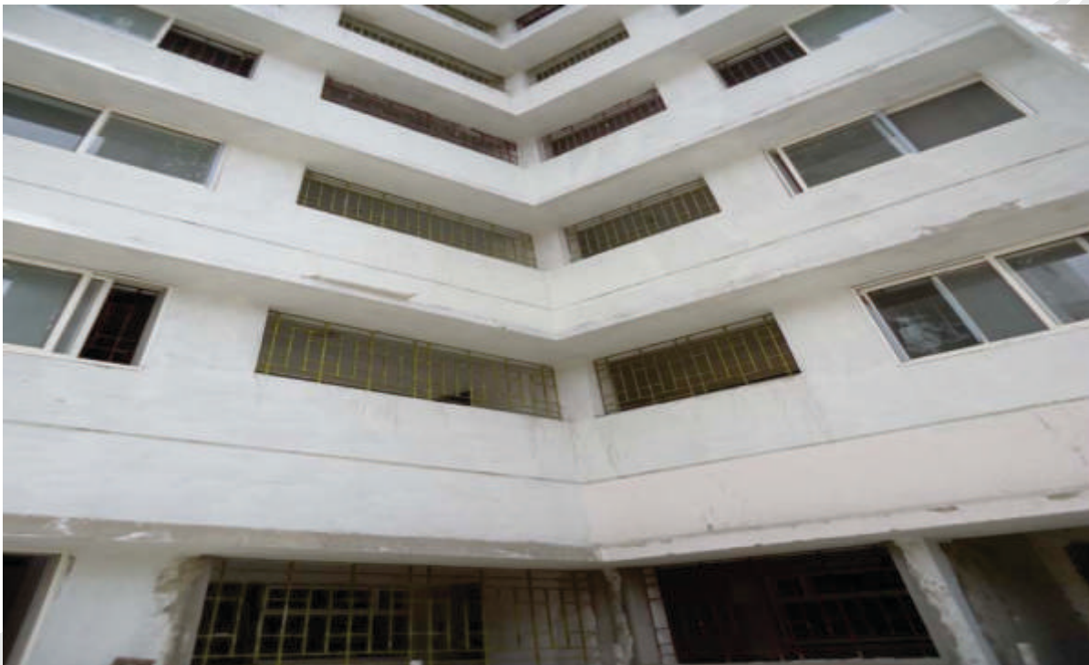
Fixing of Window, Utility grills and Aluminium windows are in progress
