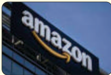
Amazon Data Center Meerkhanpet
