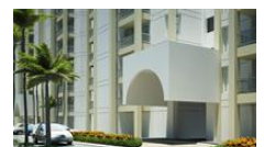
Road Side View
