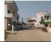
Facing Road View
