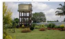
Water Storage Tank
